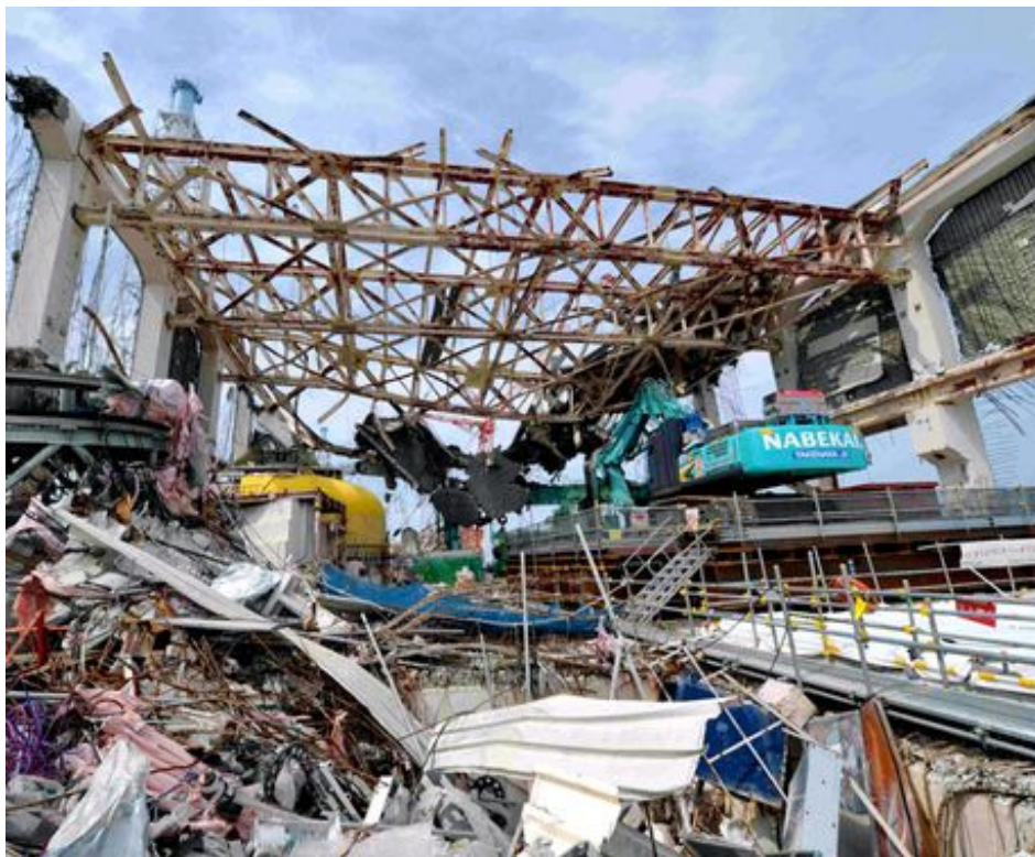
The fifth floor of the No. 4 reactor building at the Fukushima No.1 nuclear power plant as seen on May 26. The spent fuel rod pool is on the right, covered with a white tarp. (Pool)
